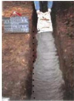
Spread GENEARTH about 3~5 cm deep on the conductor to completely cover
