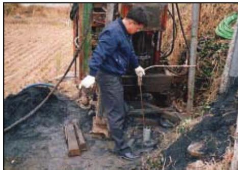
1. Auger a hole to a depth of 15cm less than the length of ground rod.
