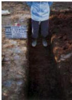
Carefully cover the GENEARTH with soil to about 10cm depth, making sure not to expose the conductor.
